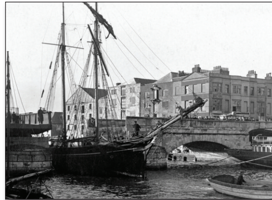
The Victorian Weymouth Bridge with a swinging central section.
