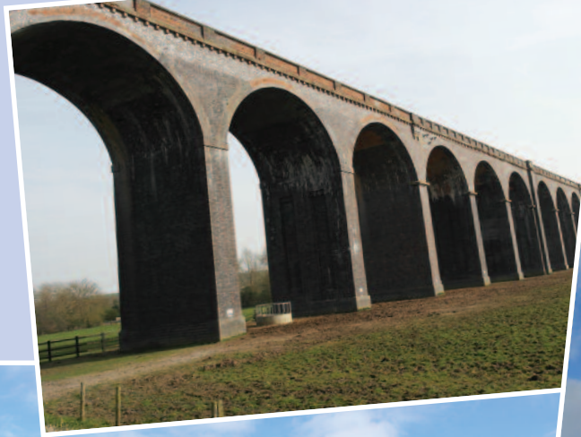
Some of the 82 arches of the amazing Harringworth (Seaton) Viaduct.
